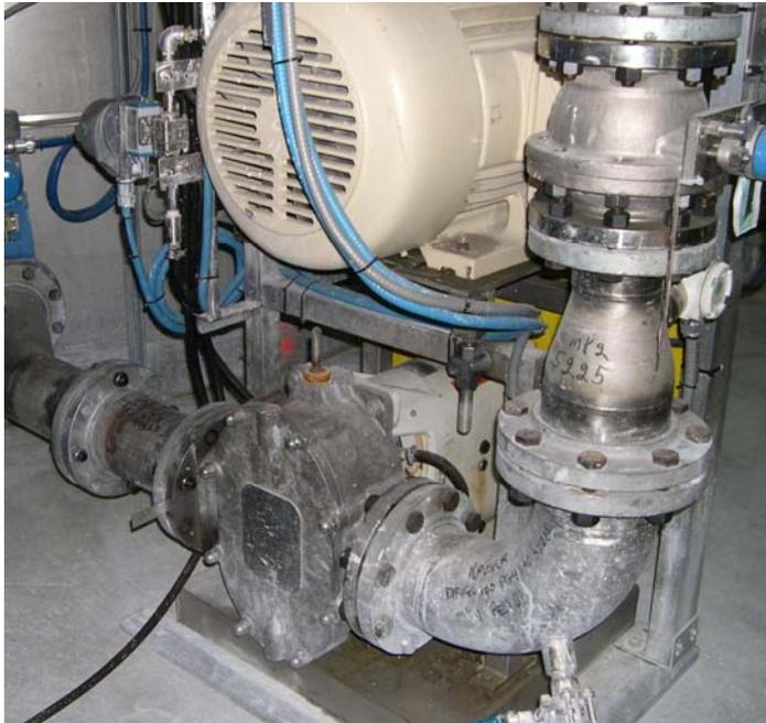
*Example of a poor installation showing a short radius bend fitted directly on to the pump discharge connection.*
